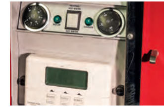
The control panel is housed behind the large, left door
