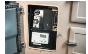
The controls and timer are housed behind the large, left door
